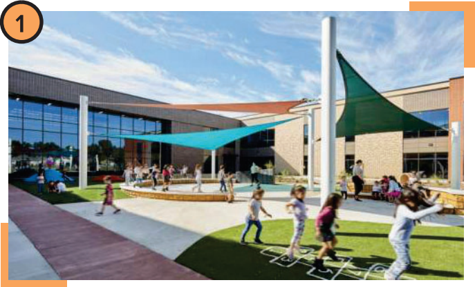
New Permanent Buildings
